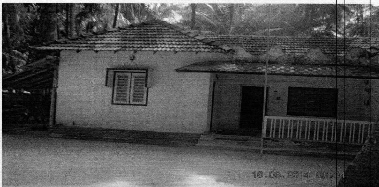
Fig 2.8: Typical Katchha house at Kavaratti Island
